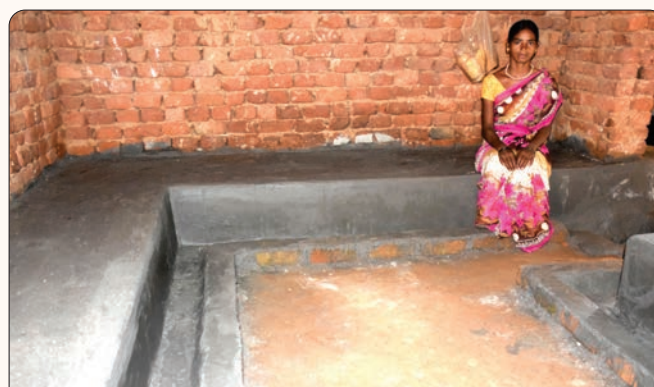
Construction of Raised Platform for Goat Farming
