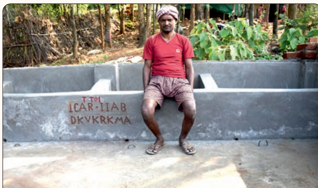
Construction of Cow Floor
